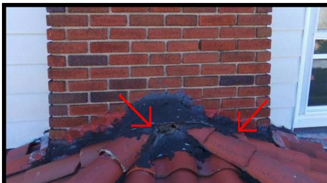
Indications of past water intrusion
