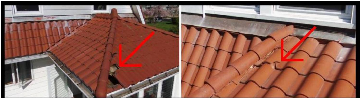
Missing tiles | Cracked tiles
