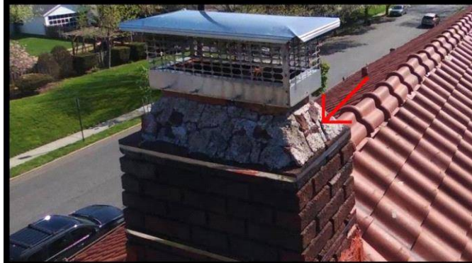
Cracking masonry
