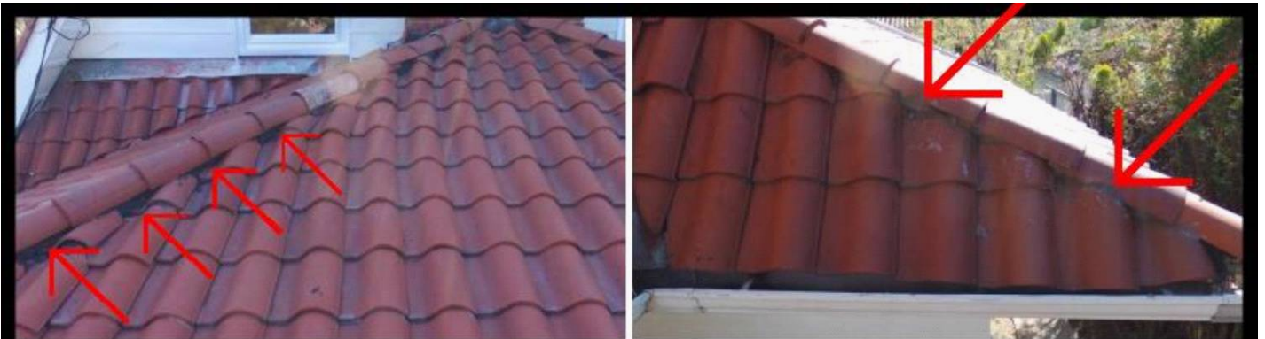
Mastic indicates prior leakage
