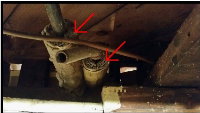
suspected asbestos
