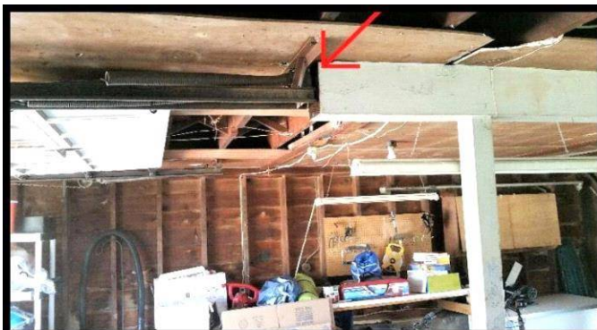
improper framing
