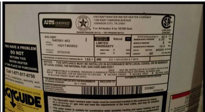
Water heater data plate
