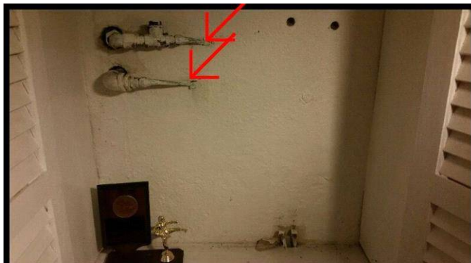
indications of a buried fuel tank
